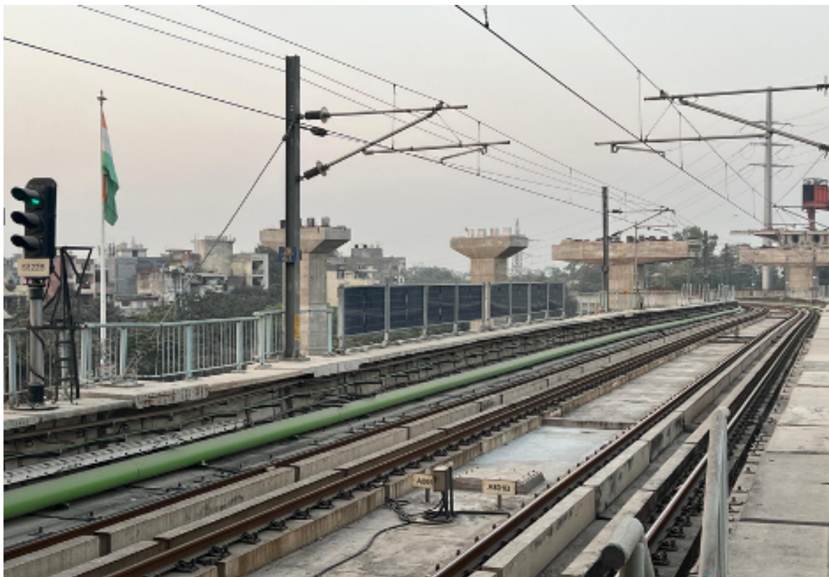
Figure 7: DMRC's trackside vertical solar pilot under construction, November 2024. Photo credit: Riding Sunbeams.
